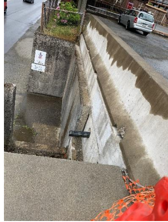
Ketchikan Bulkhead retaining driveway
